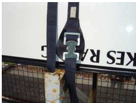
Too thin Wrong!
